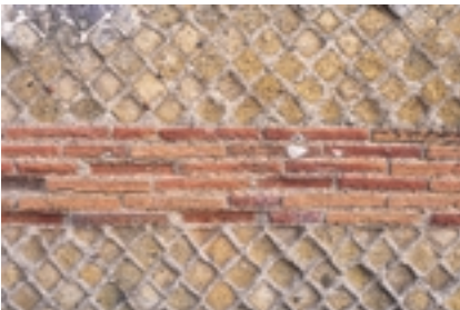
Opus reticulatum with brick layers.
